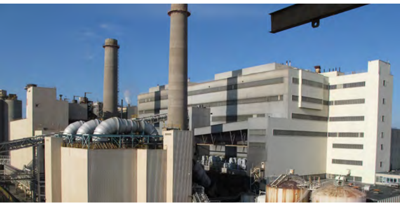
Eddystone Generating Station Units 1 and 2 before demolition, Eddystone, Pennsylvania
