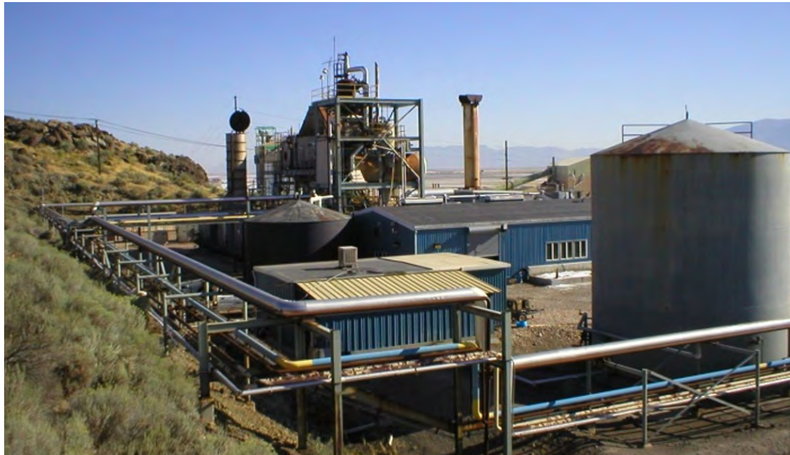
APTIM provided PacifiCorp's Little Mountain Power Plant located in Ogden Utah Decommissioning Support
