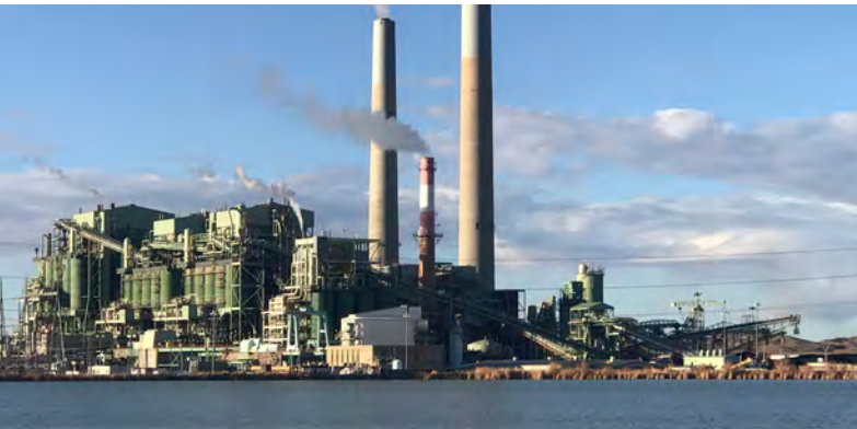
The Cholla facility is a coal-fired power plant located in northeastern Arizona
