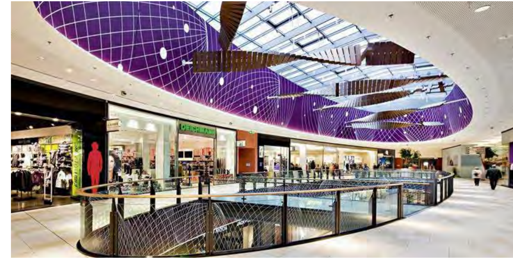
LOOP5 SHOPPING CENTER, GERMANY
