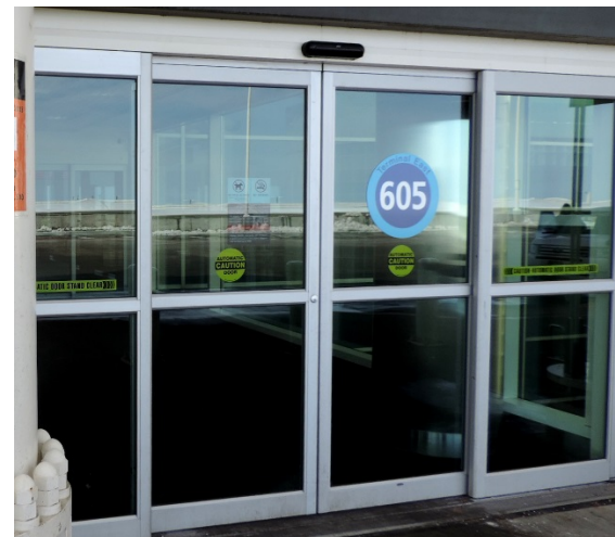
Figure 4 – East Side, Level 6 Exterior Door
