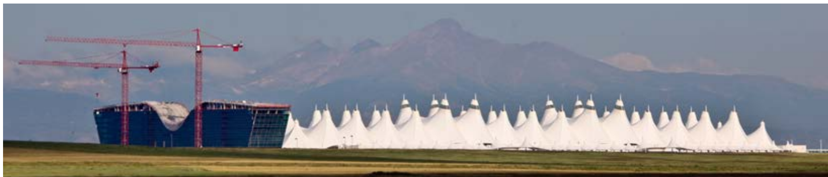
Figure 2 – DEN Terminal and Hotel
