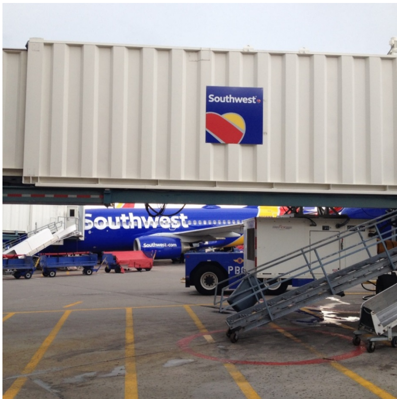
Figure 57 – Passenger Loading Bridge Signage (Exterior)
