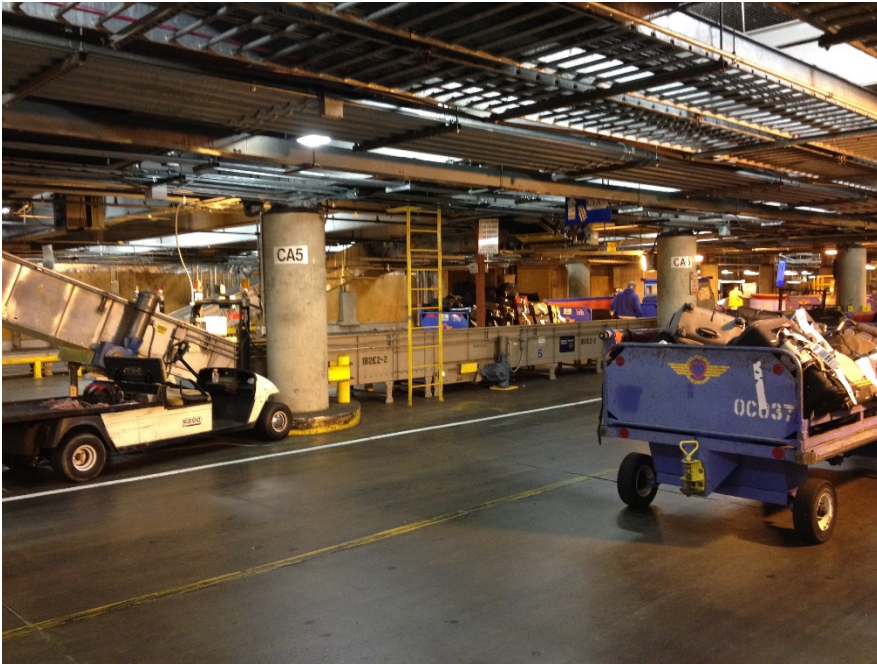
Figure 17 – Arriving Baggage Conveyors
