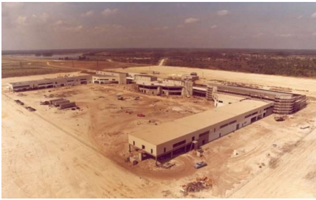
Original 1983 Terminal under construction
