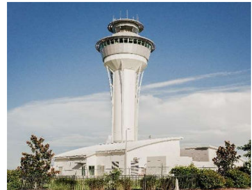
New Airport Traffic Control Tower
