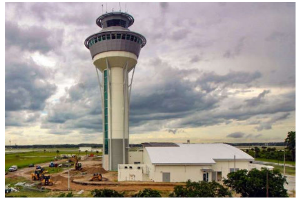
Future Airport Traffic Control Tower
