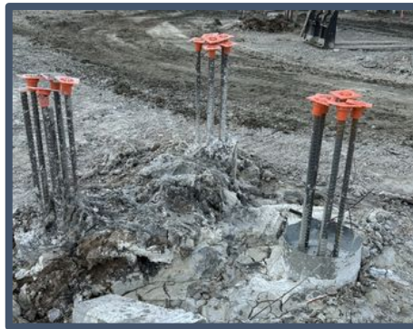
Auger Piles installation
