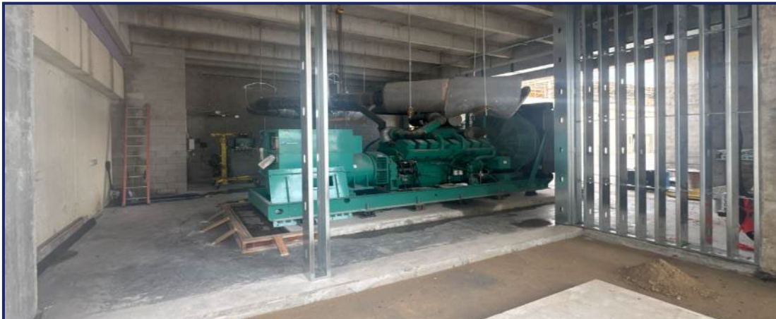
Zone 15: Generator Relocation
