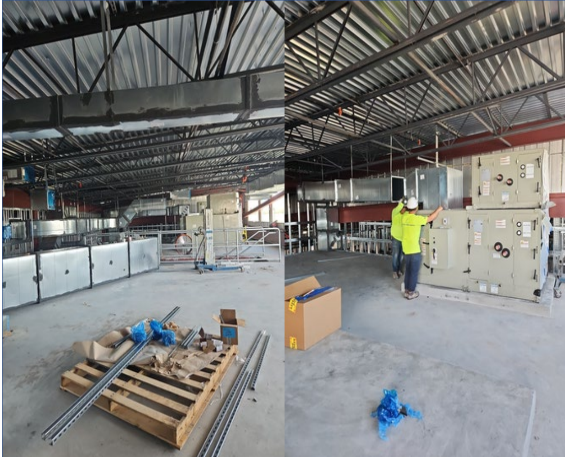
Mechanical Level Mezzanine Progress
