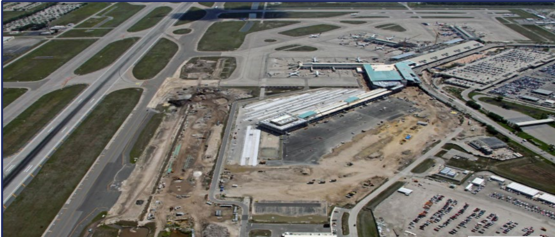
Terminal Expansion – Aerial photo of project site
