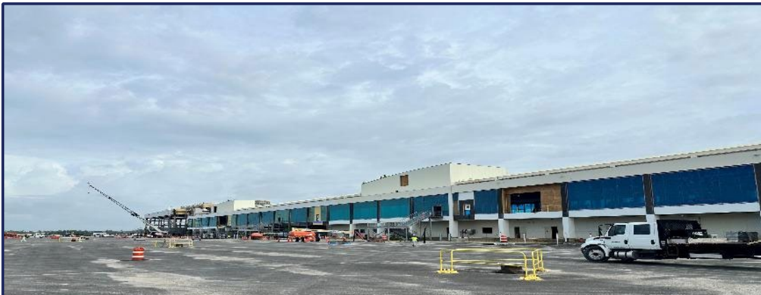
Concourse E – Facing south toward zone E3 Curtainwall installation & Exterior Stucco
