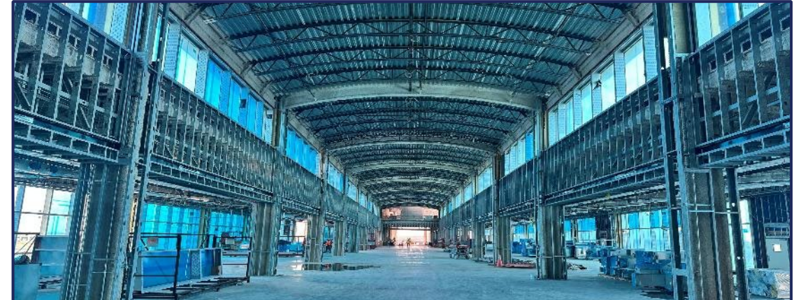
Concourse E – Curtainwall Installation and Overhead MEP throughout Departures
