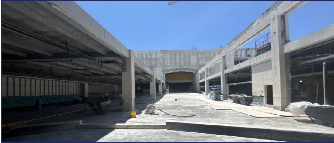
Concourse C Entrance: Demo
