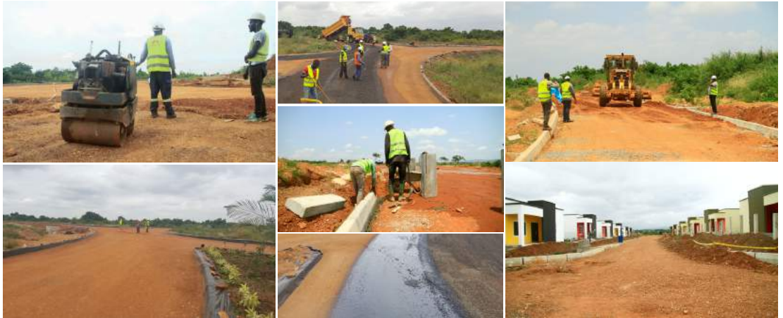
Pictures of roads under construction at Appolonia
