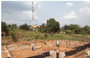
Pictures of building under construction
