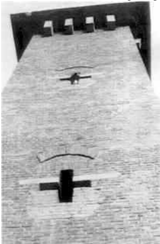
Bell tower of Orthodox cathedral Evangelismos in Tirana. Note bricks knocked out of crosses, now restored.
