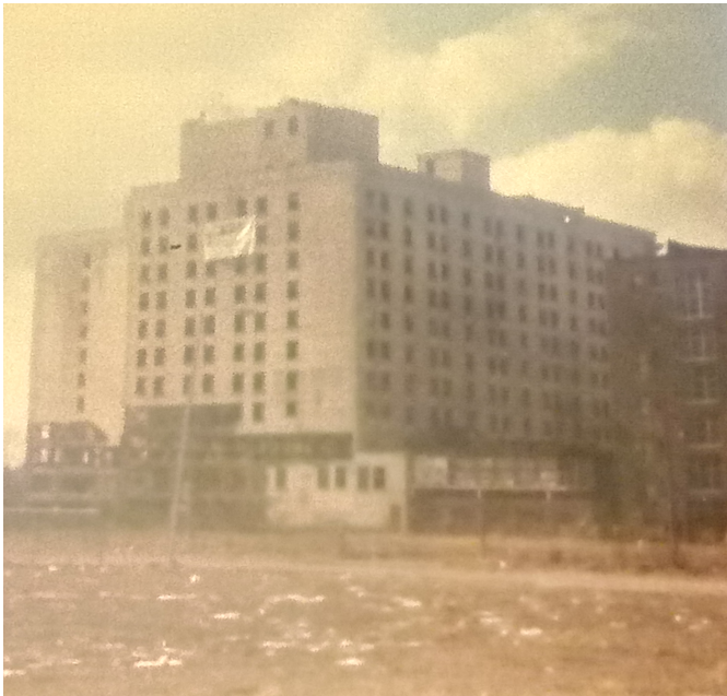
LaSalle Hotel prior to implosion
