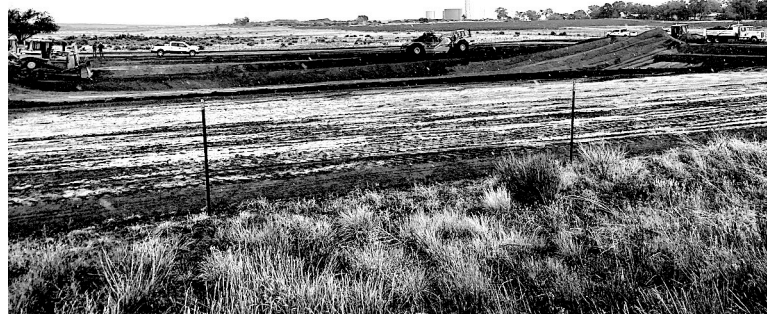
Emergency County Pond work on 7.7 road near PSC
