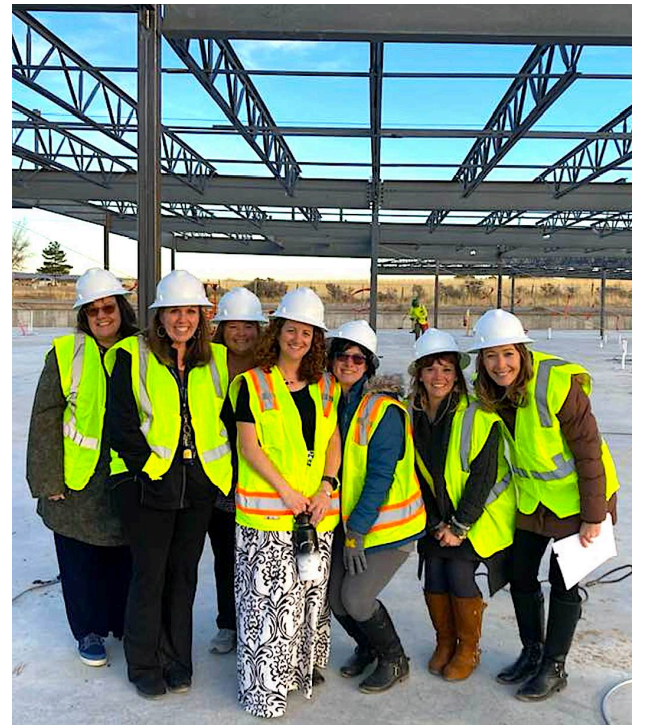
Courtesy photo 7th Street Elementary School New Building taking shape! Steel beam signing last month
