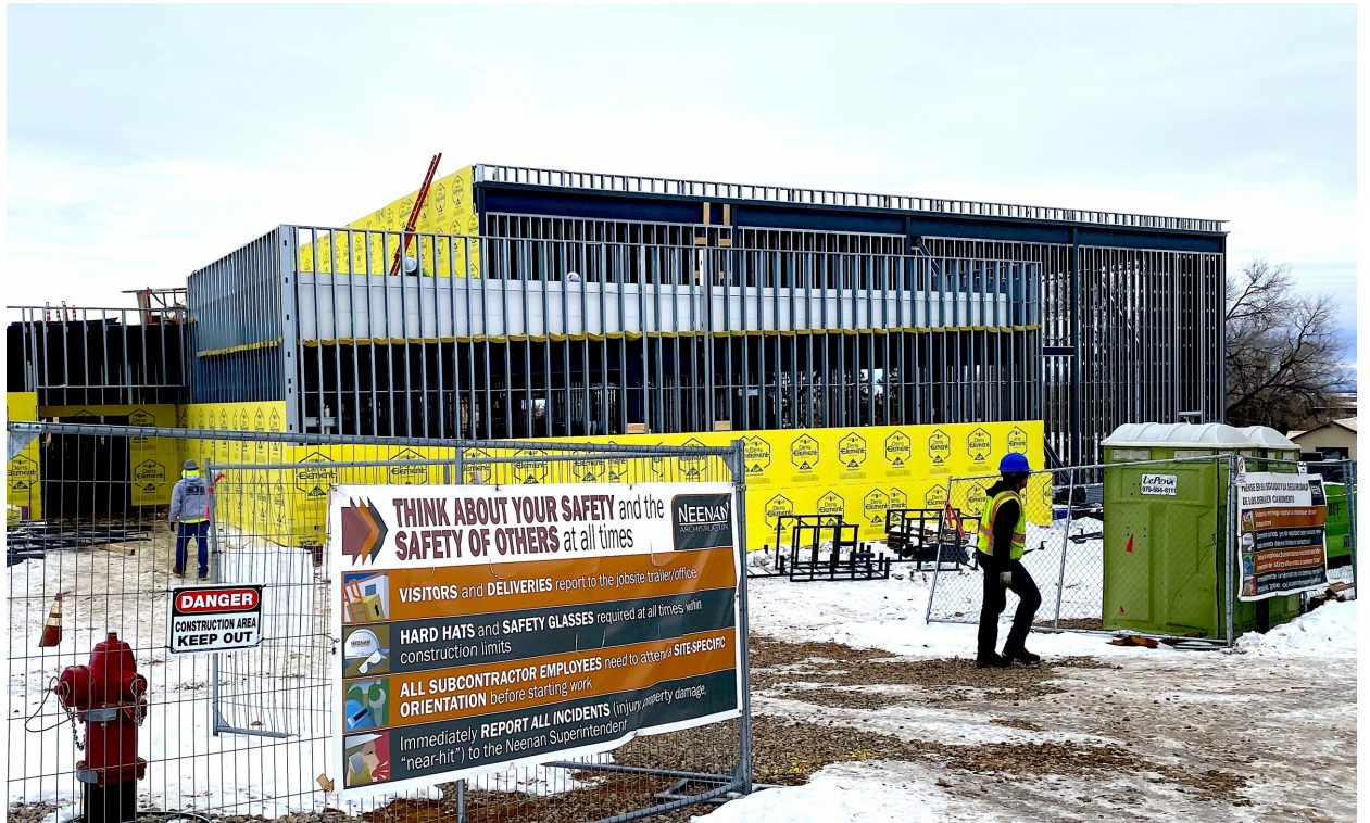
The new Elementary 7th Street School is starting to take shape
