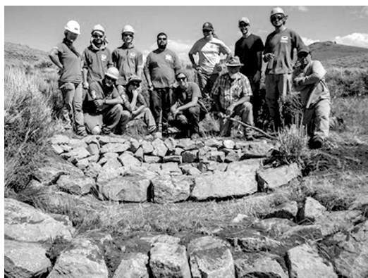
Western Colorado Conservation Corps field crew and restoration experts complete a Zuni bowl and one rock dam at Chance Gulch. Photo © Andrew Breibart, BLM (aka Zeedyk structures) Nature.org
