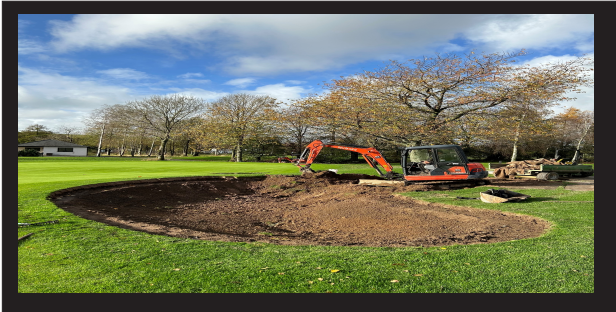
Bunker Work on the 8th
