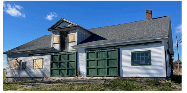
White Barn Exterior Restoration
