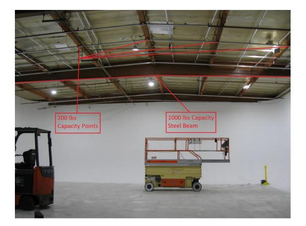
Steel Beam: Beam clamps can be used to spread loads across the beam.
